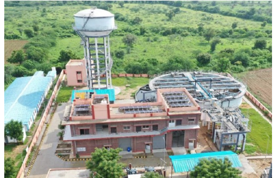
5 MLD STP Plant at Sirohi, Rajasthan from L&T Construction
